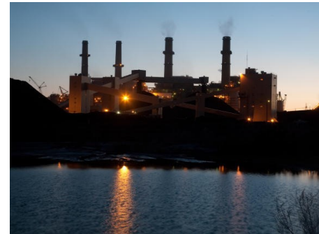
San Juan Generating Station
