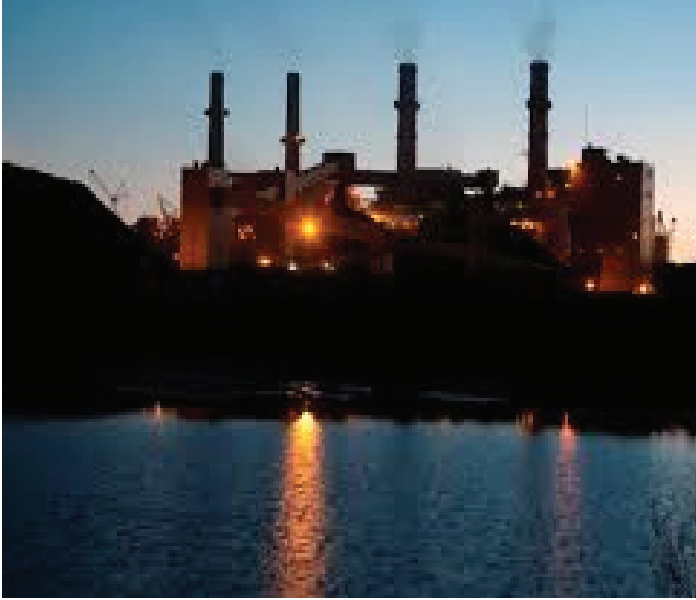
San Juan Generating Plant. Photo courtesy of the Durango Herald.
