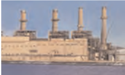
San Juan Generating Station
